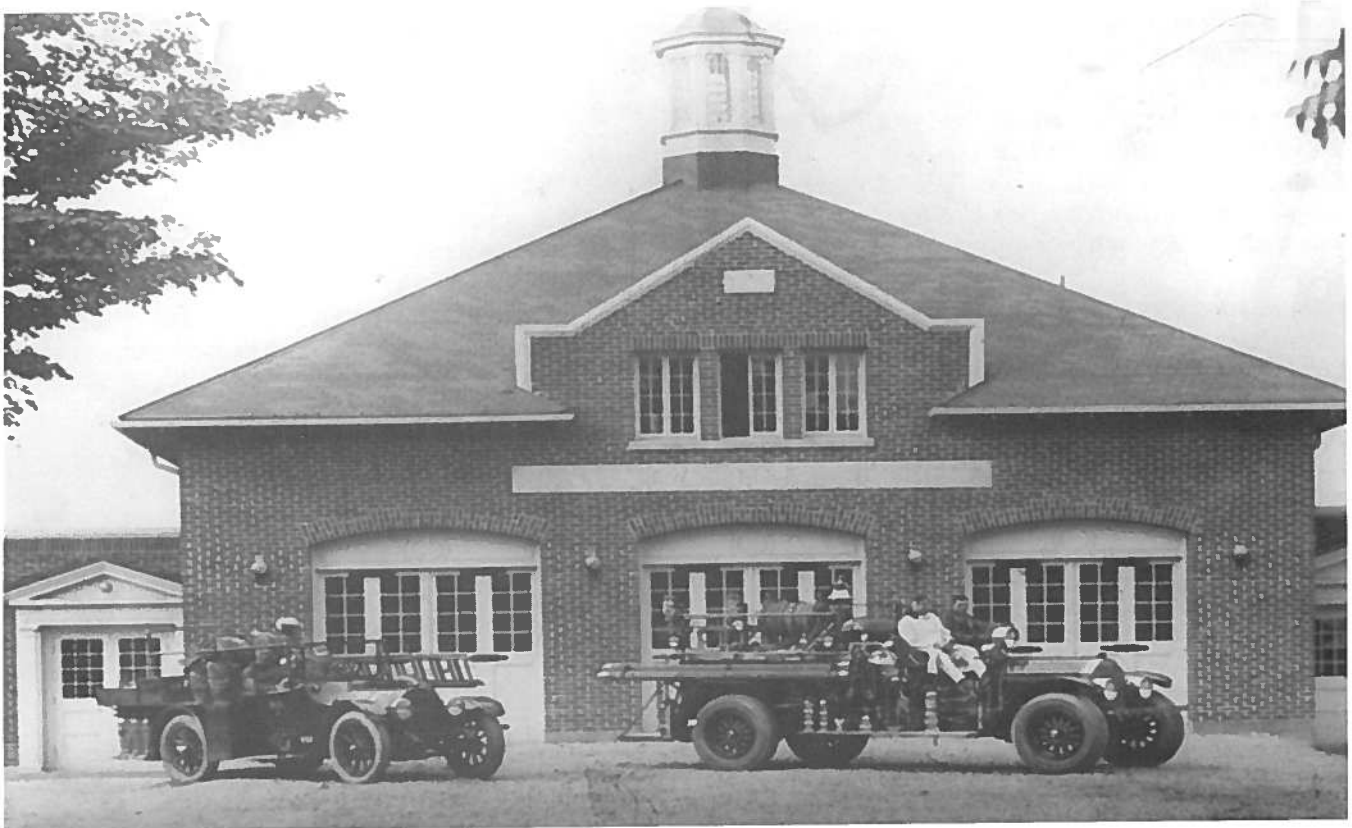
1927 Picture of Completed Lake View Fire Hall 1916 Cadillac (l.) converted into a chemical truck and 1926 American LaFrance Pumper (r.)
